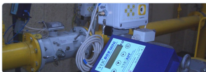
Gas metering point: VERIBOX-MINI at the volume converter
